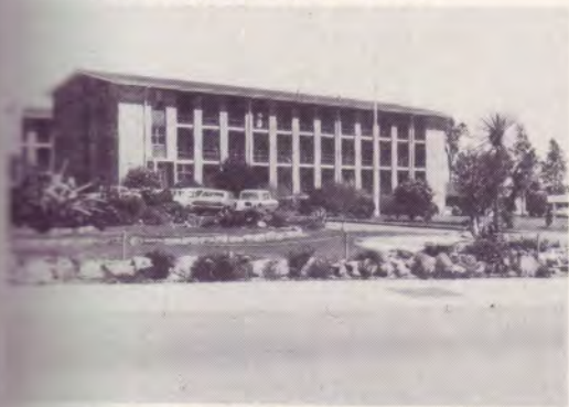
Section of the High School built in 1967.
