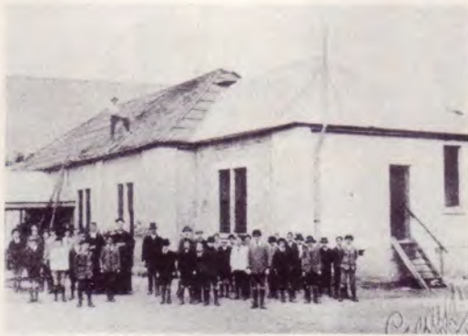
The Old School in 1918. Demolition had commenced.
